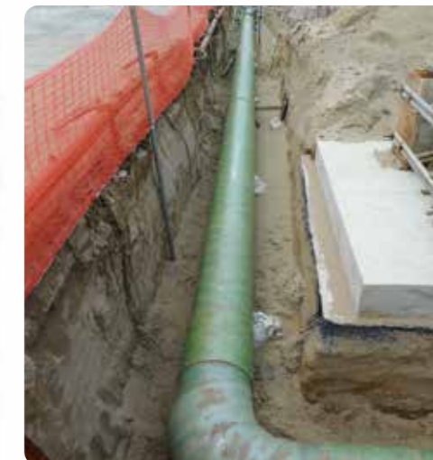
Chemical factory : drain pipe (buried)
