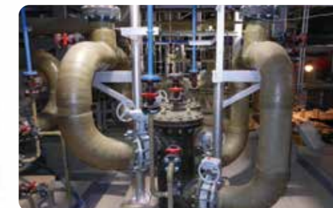
Waste incineration plant : washing water piping
