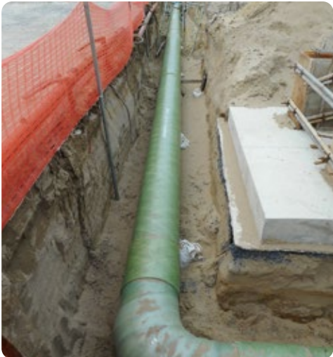
Chemical factory : drain pipe (buried)
